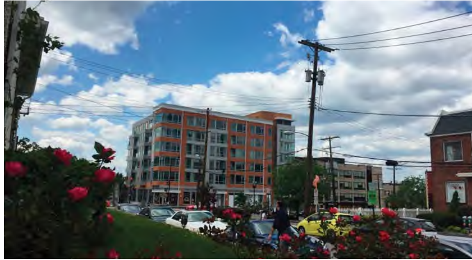
1 LOOKING NORTHWEST ACROSS WISCONSIN AVENUE
