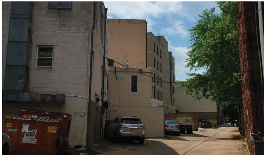
5 LOOKING SOUTH DOWN REAR ALLEY
